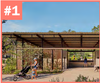
NEW RESTROOMS IN UPPER PARK
