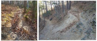
erosion that need to be addressed and water diverters that need to be cleaned out and new ones built to improve drainage.
