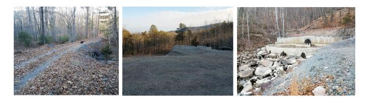
The Trough Trail: This is a 1.08-mile natural surface trail that heads west from the Timberview parking area and terminates at the Brushy Mountain Trail. It receives moderate use during spring and summer, heavy use in the fall and light use in winter. The trail is in poor condition, with a bit of water runoff and erosion. There are several water diverters that need to be cleaned out and re-established to reduce trail
