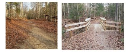
Jacobs Drop Trail: This 0.52-mile natural surface trail is part of an old fire road that connects Brushy Mountain and Kerncliff trails. The trail receives light use and is in poor condition with significant drainage issues and erosion, requiring new water diverters. Existing diverters need to be repaired, drainage ditches should be cleaned out and re-established, and a new culvert added.
