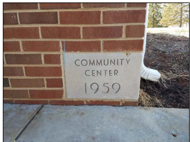
Typical Downspout Conditions
