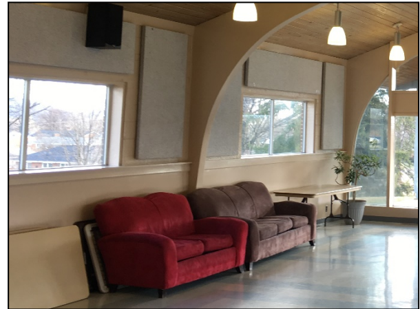
Interior Walls with Tectum Panels
