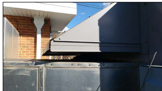
Outside Air Intake
