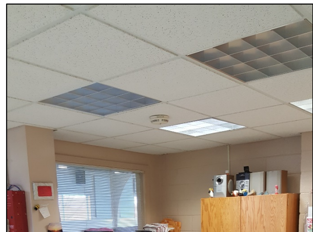
Typical ACT Ceiling
