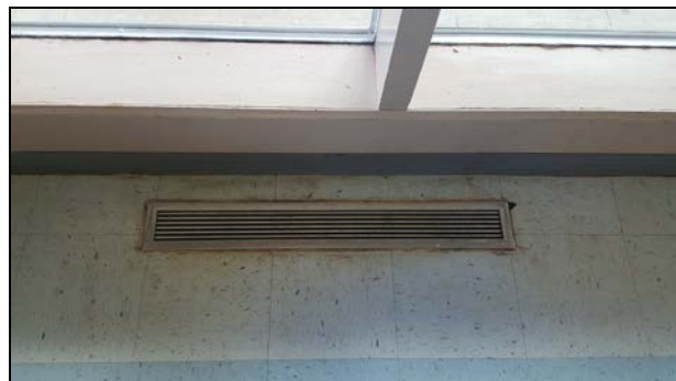
Typical Floor Register
