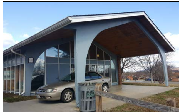
Glulam Porch and Windows
