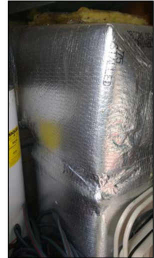
Duct Plenum to Underslab
