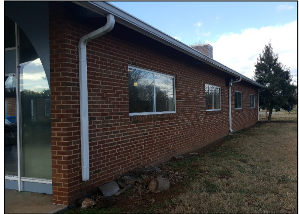
Typical Exterior Masonry
