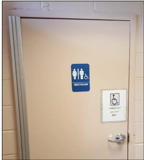
Signage at ADA Compliant Toilet
