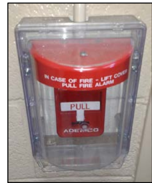
Typical Pull Station
