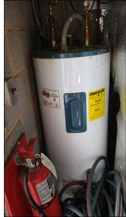
Domestic Water Heater
