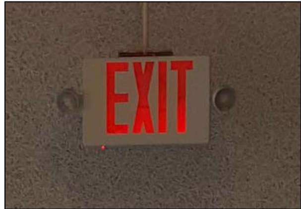
Typical Exit Sign
