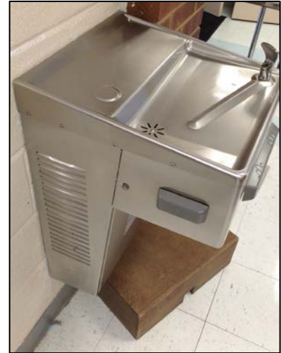
Electric Water Cooler
