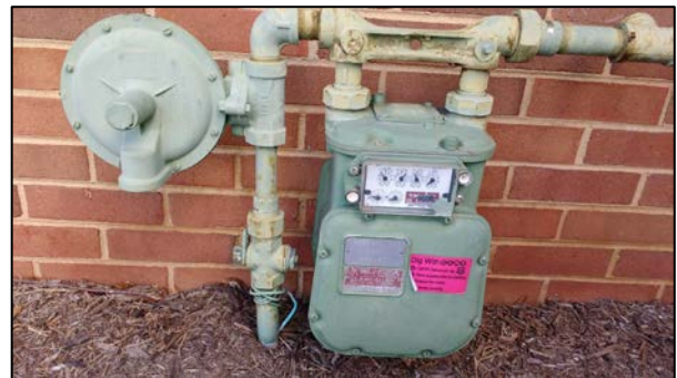
Natural Gas Meter
