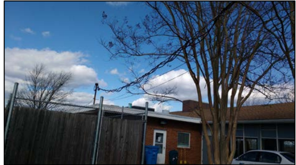
Electrical Service Entrance
