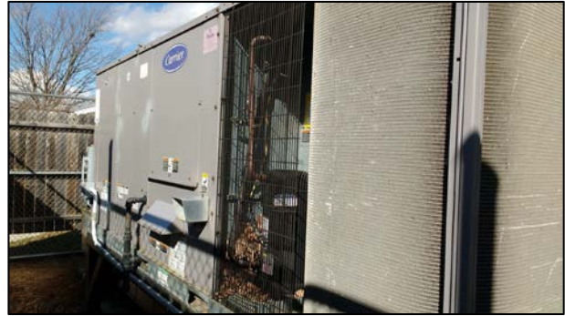
Packaged Air Handling Unit
