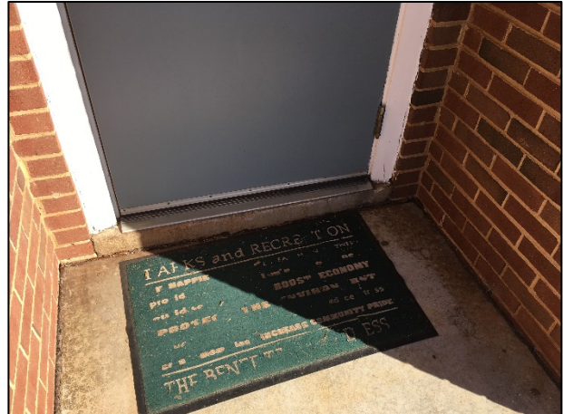
Threshold at Side Entry
