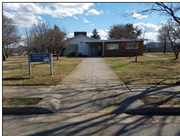
Preston Park Recreation Center
