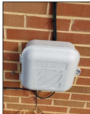
Data Service Entrance
